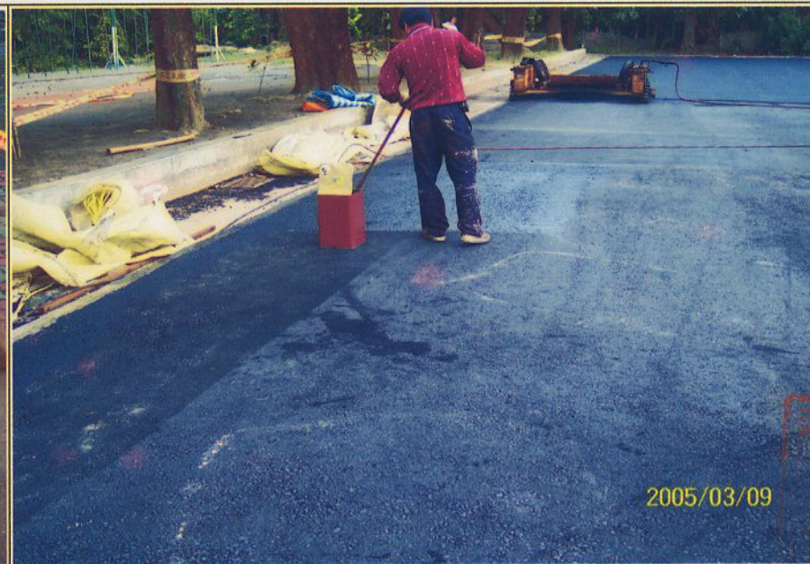
PU底漆施工塗佈
